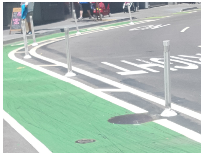
Separated Bike Lane Buffer with striping, flexible Delineators, and Green Traffic Paint.
